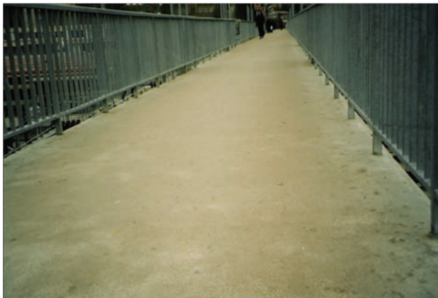
Fig 3. Polymer surfacing on footbridge deck
