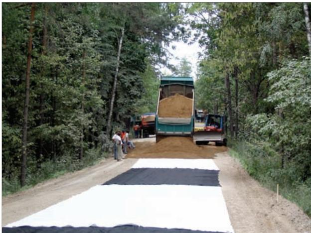
Fig 4. Geotextiles installation process
