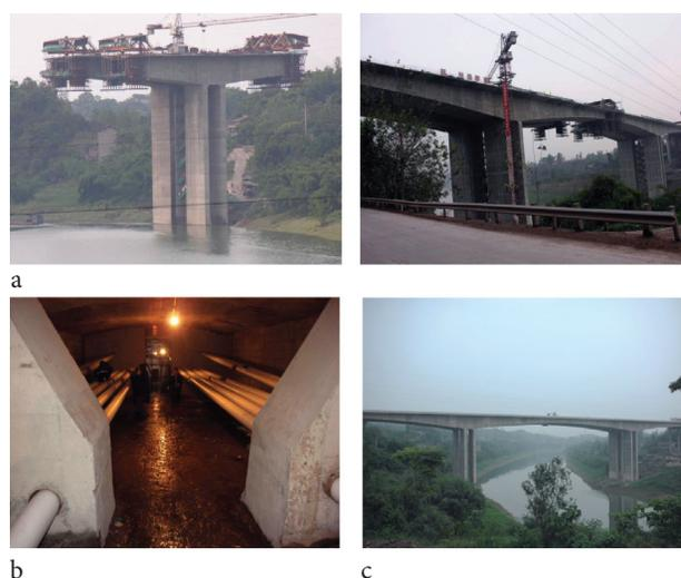
Fig. 10. Xintan Highway Bridge over the Qijiang River: a – bridge at construction stage; b – deviators and external tendons; c – longitudinal profile of bridge(from Xiaodong Guo)
