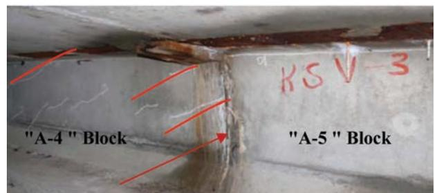
Fig. 3. Leakage in the segment joint between blocks 4 and 5
