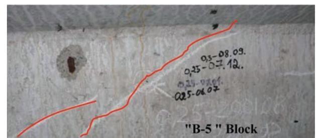
Fig. 4. Shear crack in the internal web of a box girder
