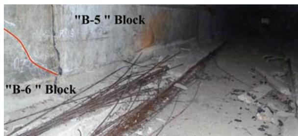
Fig. 6. The view of wires in the places of crack opening
