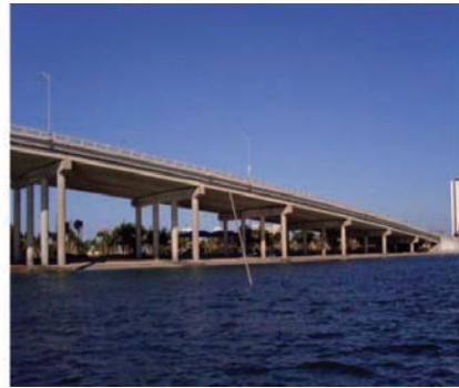
Bridge pier shafts
