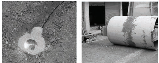
Fig. 2. 200 mm diameter pressure gauge and roller compactor compacting the subbase layer
