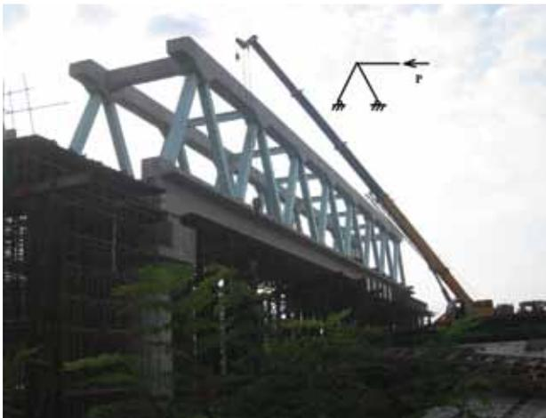
Fig. 1. Steel structure of composite truss bridge
