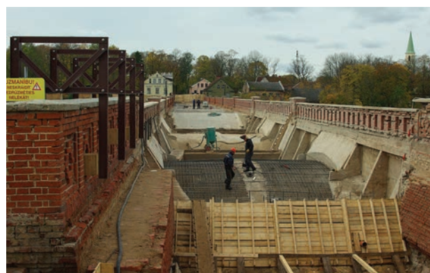
Fig. 11. Strengthening of the reinforced concrete arch span
