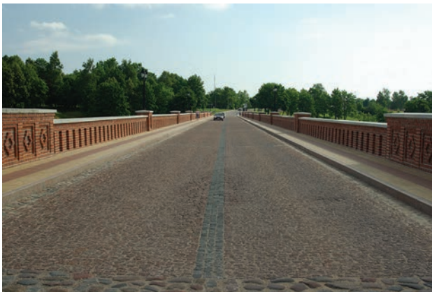
Fig. 14. Side view of the bridge after reconstruction
