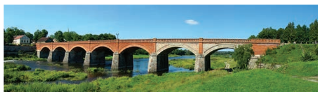
Fig. 1. Side view of the bridge before reconstruction
