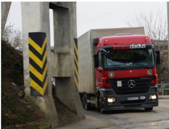
Fig. 6. Example of the bridge with insufficient lateral under-clearance
