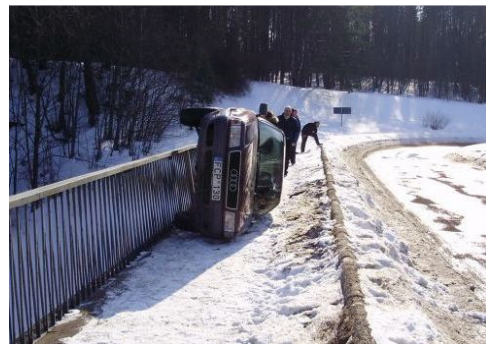
Fig. 8. Car accident on the bridge built on sharp street bend and insufficient parapet height (photo from Delphi)
