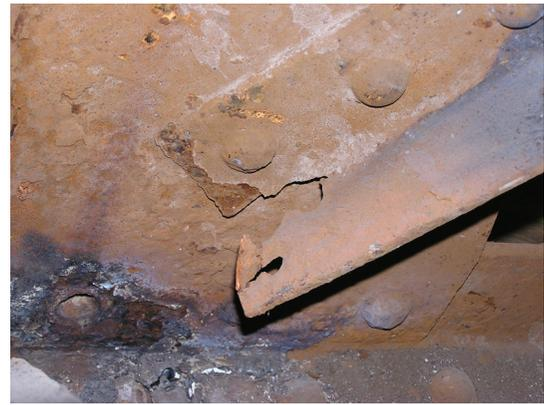
Fig. 5. A severely corroded railway bridge element
