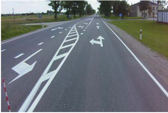
Fig. 2. Intersection with the minor road equipped with the left-turn deceleration and waiting lane
