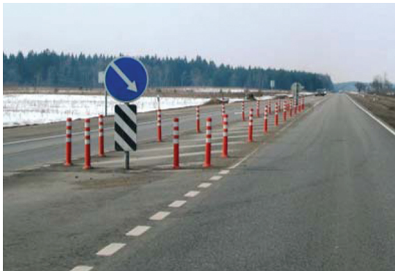
Fig. 5. Plastic reflective posts on the intersection of the road A16 Vilnius–Marijampolė
