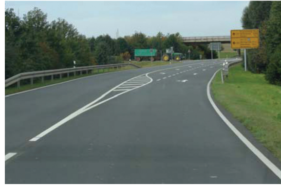
Fig. 2. Intersection with the minor road equipped with the left-turn deceleration and waiting lane
