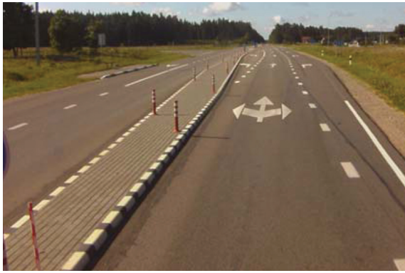
Fig. 4. Raised splitter islands in 47.88 km and 61.14 km of the main road A11 Šiauliai–Palanga
