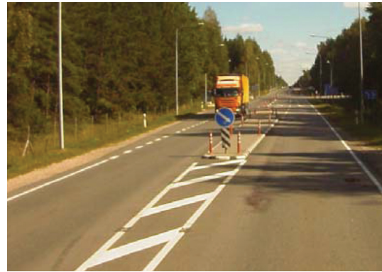
Fig. 4. Raised splitter islands in 47.88 km and 61.14 km of the main road A11 Šiauliai–Palanga
