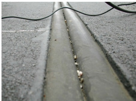
Fig. 4. The bridge movement joint on Bridge A
