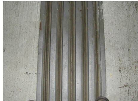
Fig. 6. The bridge movement joint on Bridge B
