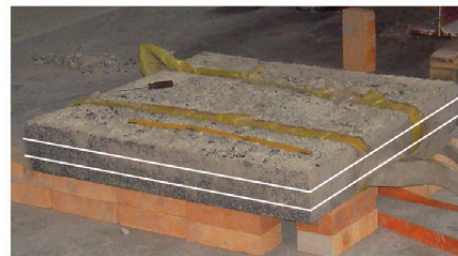
Photo of example 1x1 m specimen cut-out from pavement
