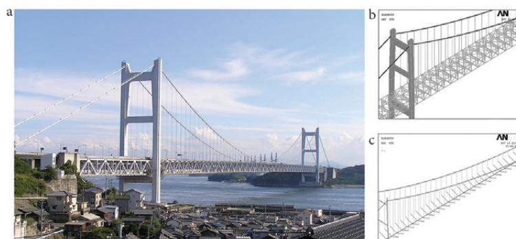
**Fig. 1.** The structure and FE models : a – Shimotsui-Seto suspension bridge (by Tatushin, September 2008; with permission); b – detailed bridge model for matching the real modal characteristics; c – validated simplified bridge model used in the analyses
