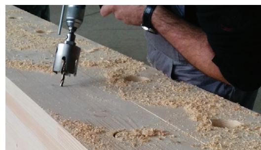
Fig. 2. Slot preparation for the CHS inserts
