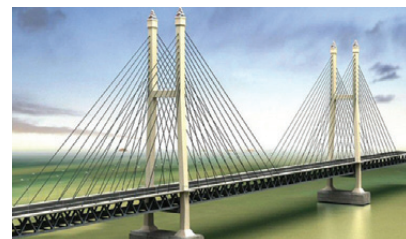
Fig. 3. Cable-stayed bridge with trussed deck
