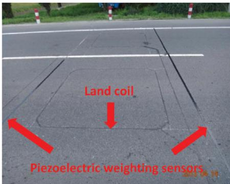
Fig. 2. Installation of WIM system
