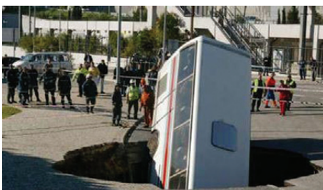
Fig. 1. Road pavement collapse with a swallowed bus
