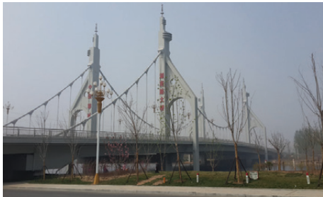
Fig. 4. Picture of Hunan Road Bridge
