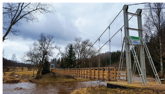
Fig. 1. Pedestrian suspension bridge over Amata River (Latvia)
