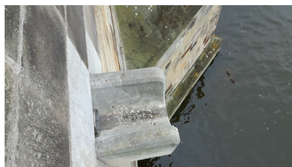
Fig. 4. Gargoyle with the new drainage system outlet
