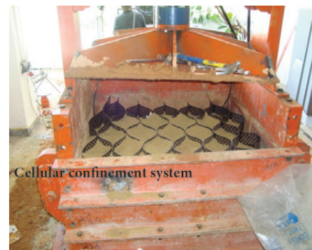
Figure 6. Confinement cells placed on the base soil were filled with sand
