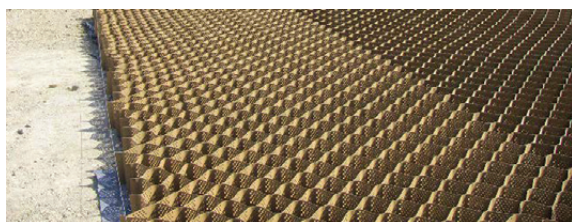
Figure 4. Application of cellular confinement system in the field (Ankara, Turkey)
