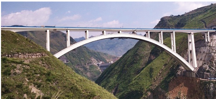
Figure 1. Overview of Beipanjiang Bridge
