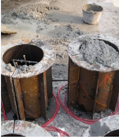
a) casting concrete
