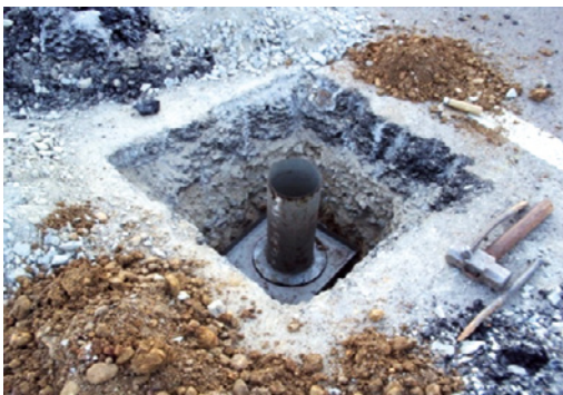
Figure 4. Observation of test pits
