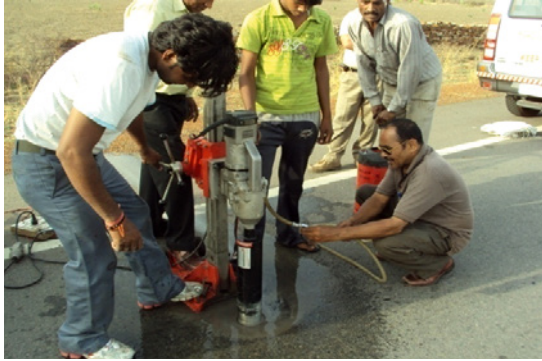
Figure 6. Full-depth core cutting of bituminous layers
