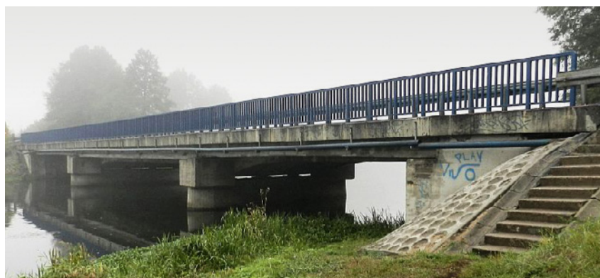
Figure 1. General view of the analysed bridge (photo A. Madaj)
