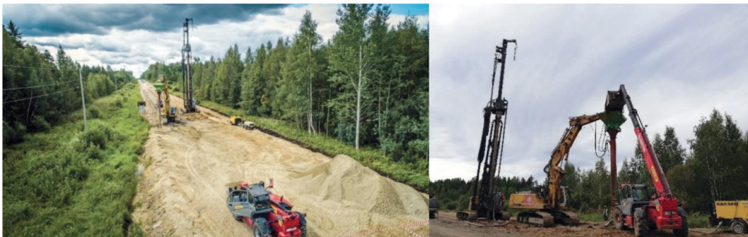
Figure 2. Construction of combined columns and pile columns
