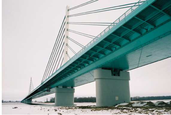
Figure 3. General view of the bridge
