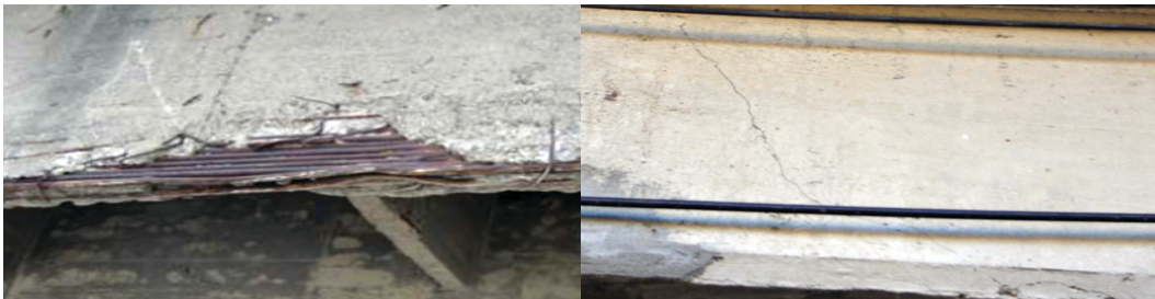
(a) Dense reinforcement
