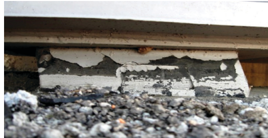
(c) Offset on elastomeric bearing
