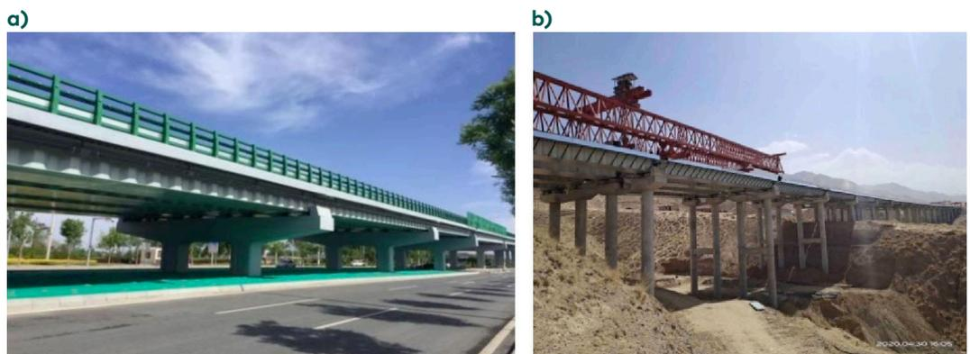
**Figure 1.** CW-SBS composite box girder at Gansu Province in China: (a) Terminal 2 connecting line continuous beam bridge at Zhongchuan Airport, (b) the construction of Dunhuang to Dangjin mountain Expressway bridge
