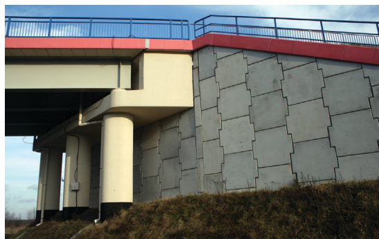
Figure 2. View of the facade elements of the abutment retaining structure
