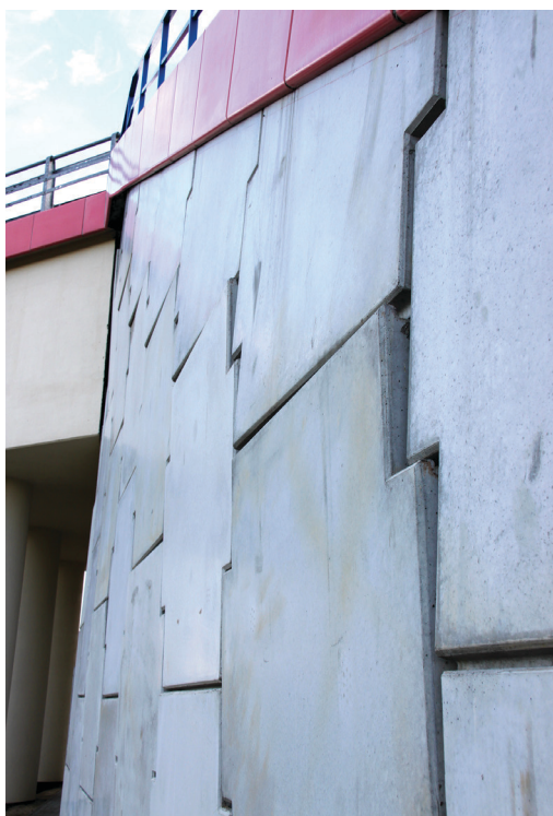
Figure 3. Selected shape defect of retaining structure surface
