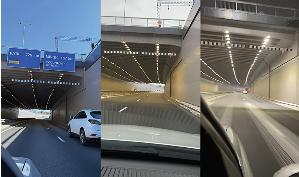
Figure 5. Liepkalnis tunnel lighting at different times (from left to right: sunny, cloudy and night)
