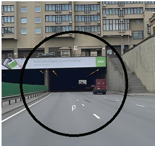
Figure 15. Gelezinio Vilko St. view of the tunnel portal from the southern side with a 20° field of view and individual parts of the field
