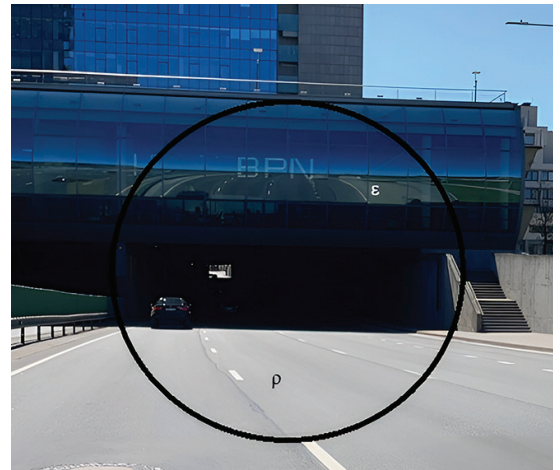
Figure 16. Gelezinio Vilko St. view of the tunnel portal from the north side with a 20° field of view and individual parts of the field
