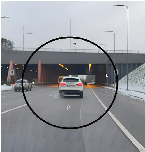
Figure 11. View of the portal of Gudeliai tunnel from the south side with a 20° field of view and individual parts of the field
