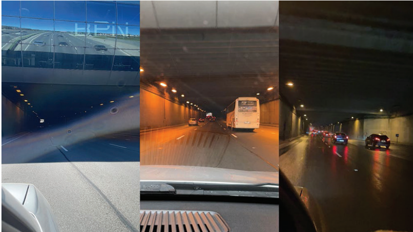
Figure 9. Geležinio Vilko street tunnel lighting under different conditions (from left to right: sunny, cloudy and night)
