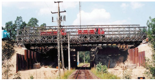
Figure 2. Diversion road with MS 22-80 bridge
