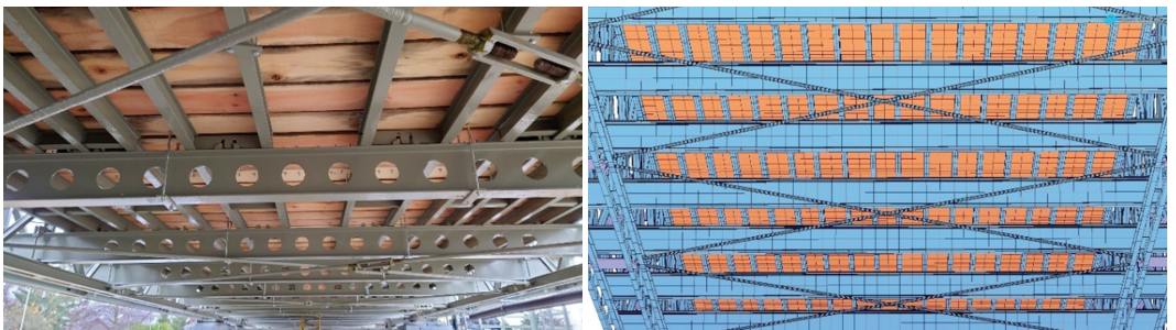
Figure 20. Bridge detail compared with the FEM model – bottom view on transoms, bracings, stringers, and platform deck
