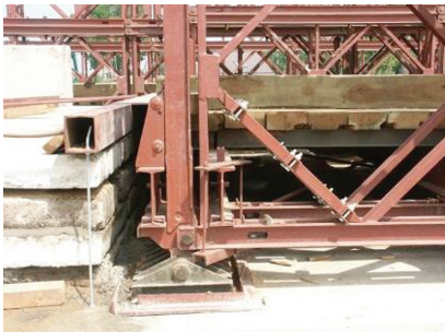
Figure 7. Bridge MS 22-80 type – different variants of fastening the crossbars to the bottom chords of panels
