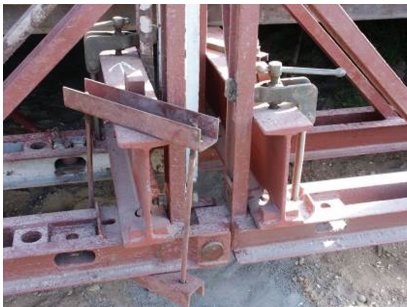
Figure 7. Bridge MS 22-80 type – different variants of fastening the crossbars to the bottom chords of panels
