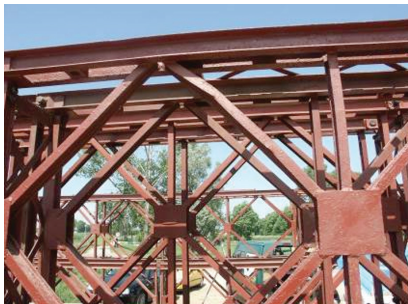
Figure 7. Bridge MS 22-80 type – different variants of fastening the crossbars to the bottom chords of panels
