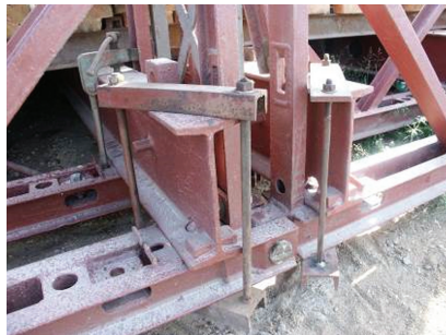
Figure 7. Bridge MS 22-80 type – different variants of fastening the crossbars to the bottom chords of panels
