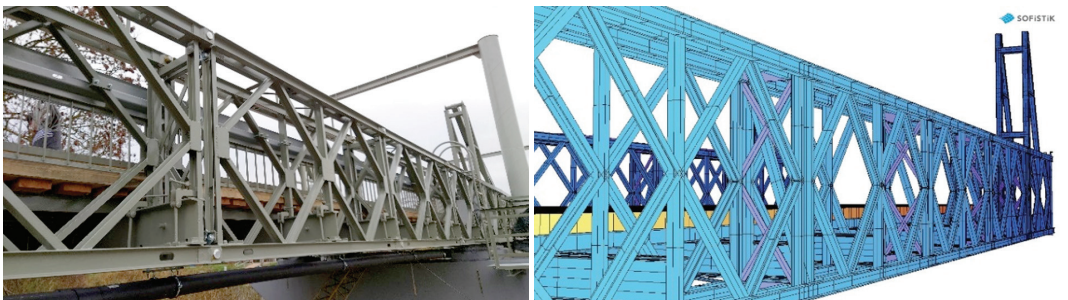
Figure 19. Bridge detail compared with the FEM model – side view of the bridge
