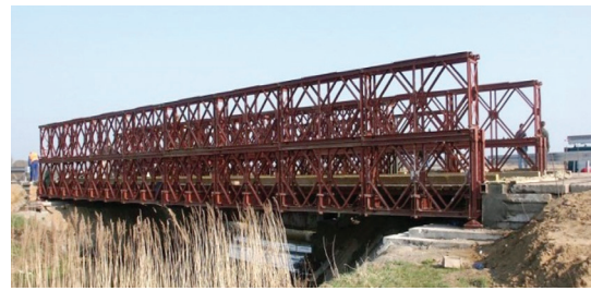
Figure 2. Diversion road with MS 22-80 bridge
