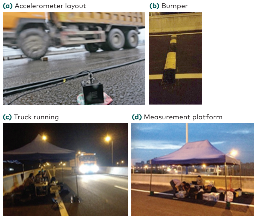
Figure 8. Details of dynamic loading test
