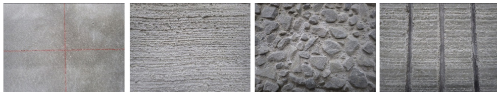
Figure 10. Surfaces of concrete pavement, trowel-finished, broom-finished, exposed-aggregate, and longitudinal groove
