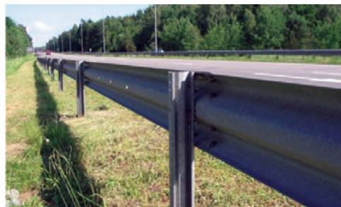
Fig. 1. Metal safety barriers without inserts used in Lithuania, meeting the safety requirements of European Standard EN 1317
